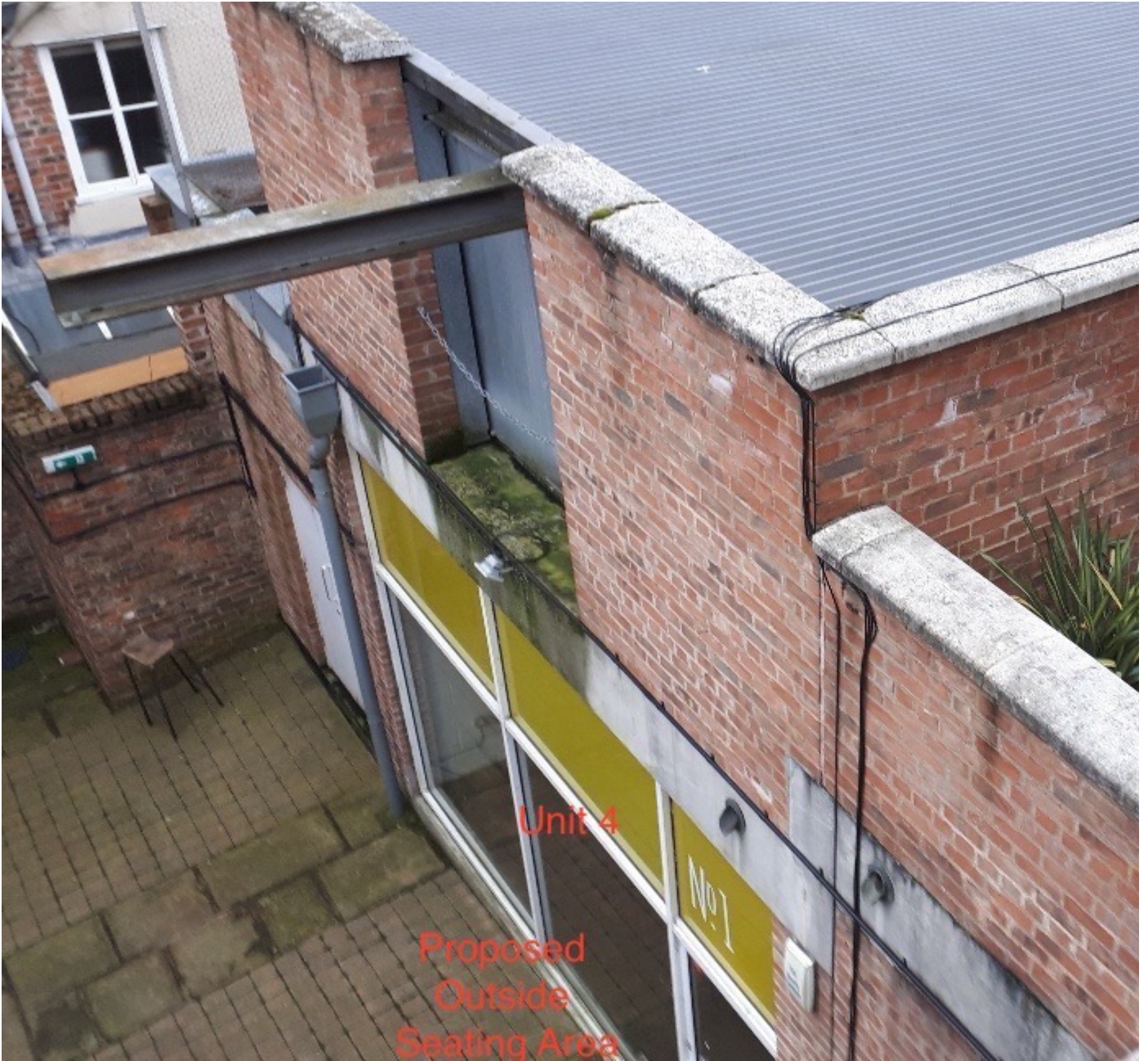
Another photo showing the proximity of Apartment 17's terrace to proposed Restaurant.
